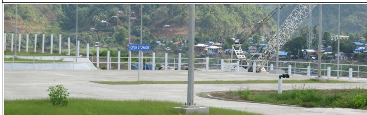
Open Storage Area
