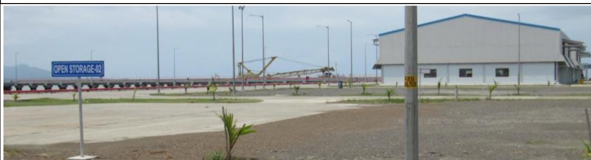
Open Storage Area
