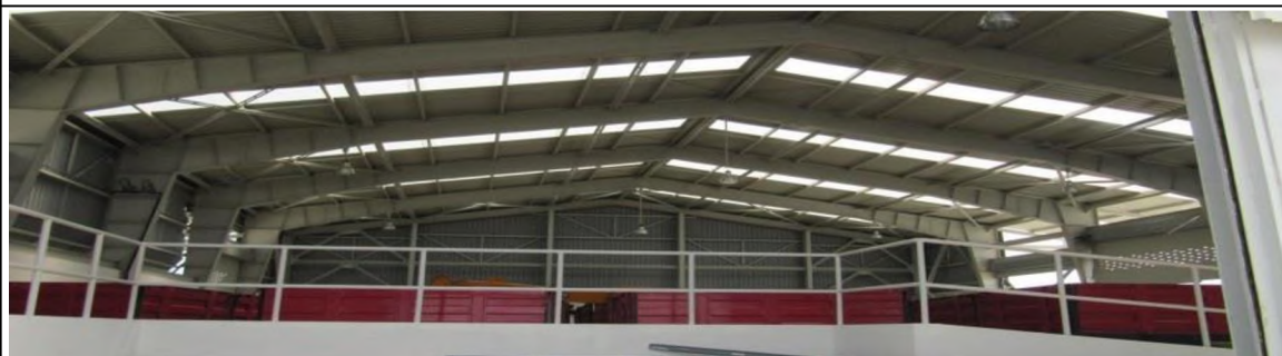
Inside view of the Covered Shed at Sittwe
